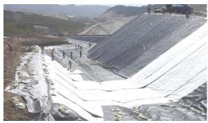
The Phase V-D project also included approximately 2.5 million cubic yards of excavation and installation of a composite liner system consisting of a low permeable layer overlain with a GCL encapsulated between a 40 mil and 60 mil HDPE geomembrane. The project also included significant perimeter drainage improvements, an asphalt concrete access road, and re-vegetation of the adjacent slopes. Rich Huffmire served as the Construction Manager on this project.
