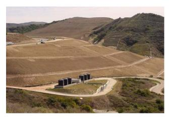
Tetra Tech BAS provided construction management for the Phase VD Groundwater Protection and Front Face Closure Project at Frank R. Bowerman Landfill. The project included construction of a partial final closure demonstration fill on the front face of the landfill. The demonstration fill provided a model for future site closures and included installation of moisture monitoring probes for testing the efficiency of the probes for testing the efficiency of the alternative soil cover.
