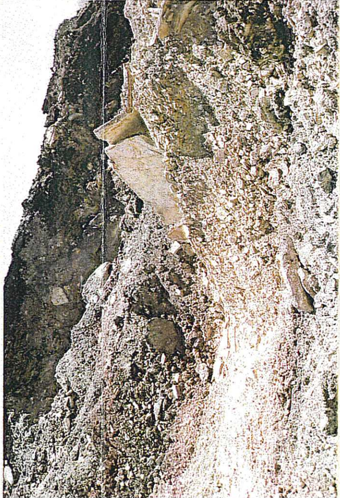
PHOTO NO. 3 EXPOSED ROCK AREA
