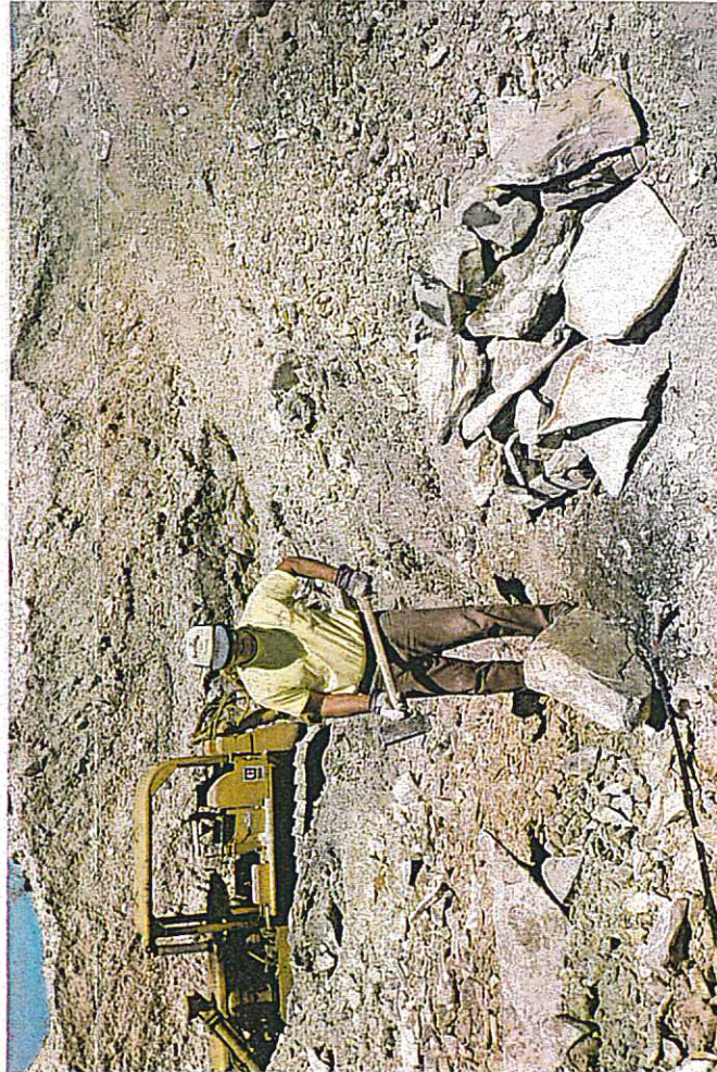
PHOTO NO. 5 HAND SPLITTING SHALE
