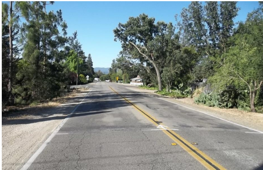
Typical road bed to be resurfaced
