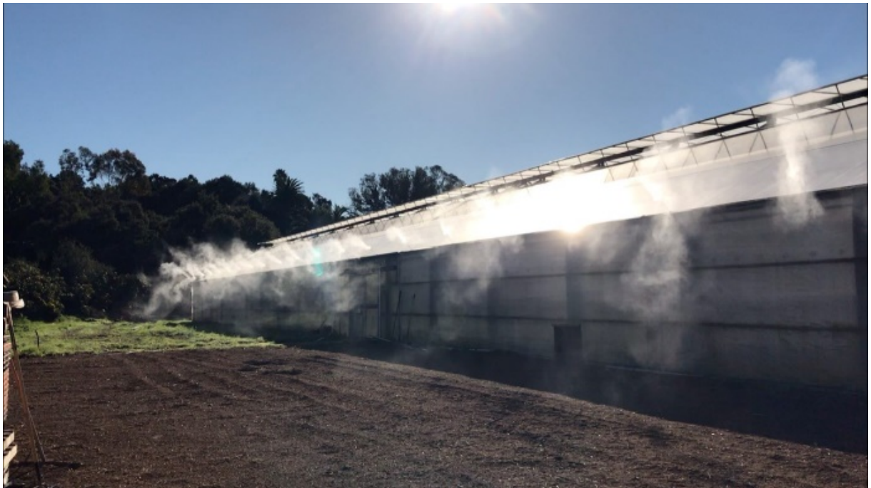
ODOR CONTROL ON NORTH SIDE OF THE “CONLEY” GREENHOUSE AT CERES FARMS
