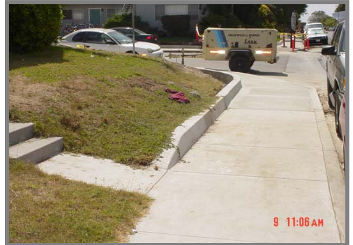
Figure 2: New sidewalk and curb ramp at 850 Cordoba
