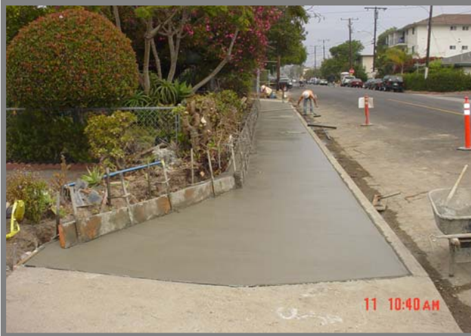
Figure 1: Fresh concrete on Camino Pescadero
