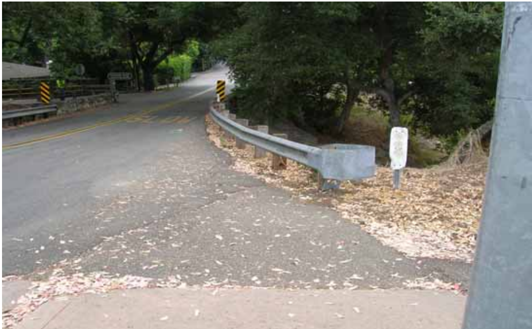
Photo: Existing Santa Rosa Lane Bridge (No. 51C-045) over Oak Creek looking east along proposed pedestrian bridge alignment.
