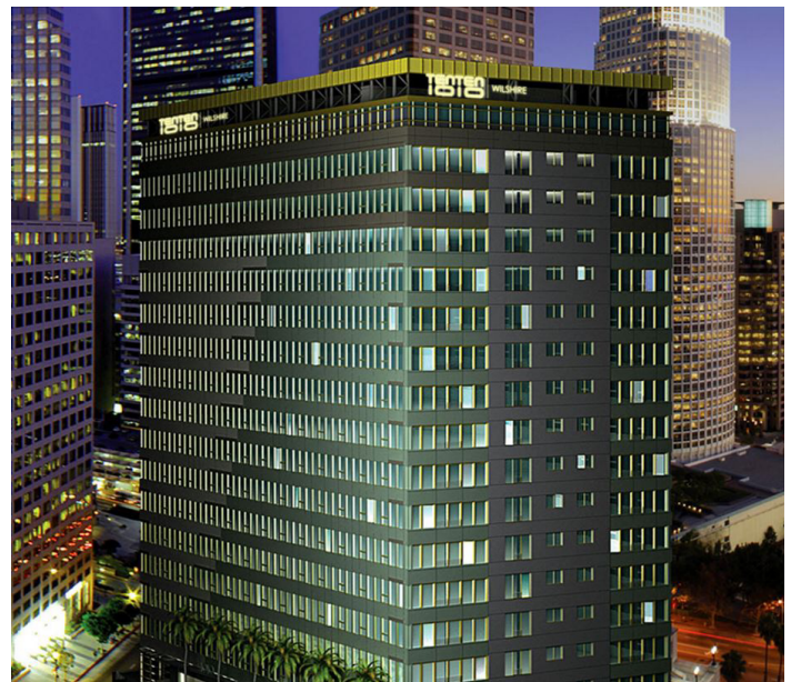
Exterior shot of 1010 Wilshire from the leasing company’s home page.
