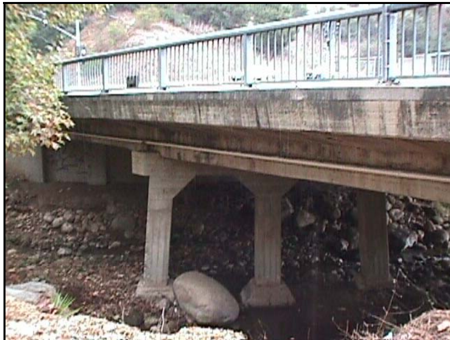
Photo: Existing upstream 1931 structure being replaced.
