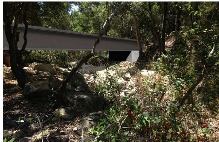
Toro Canyon Bridge
