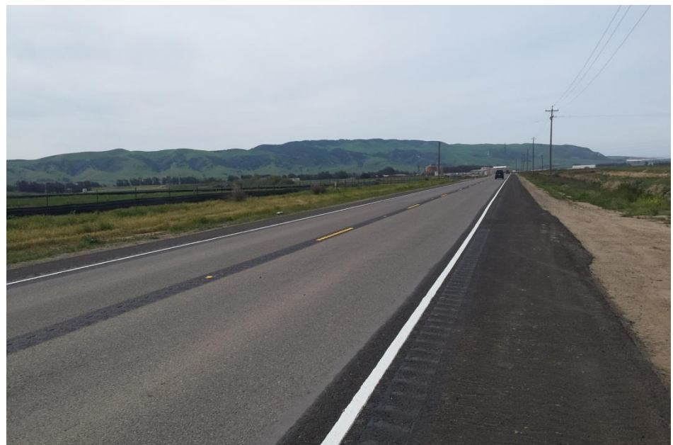
Post-construction – Betteravia Road
