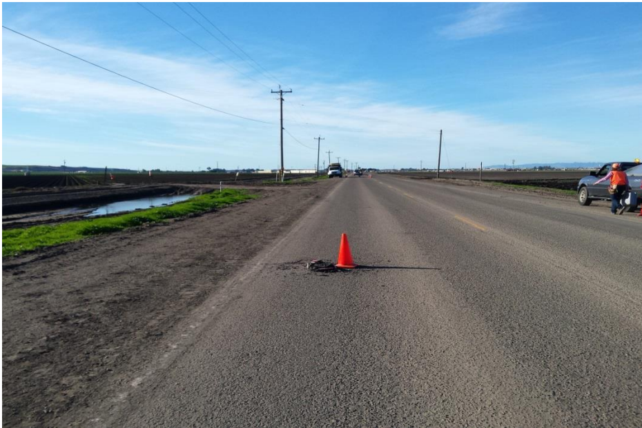
Pre-construction – Betteravia Road
