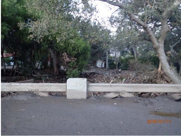
Buena Vista Creek at 192 looking upstream, bridge has since been opened.
