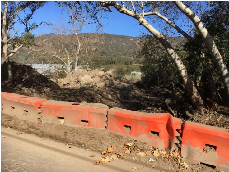
Arroyo Paridon Creek upstream of CA 192 (Bridge opened by Caltrans and County)
