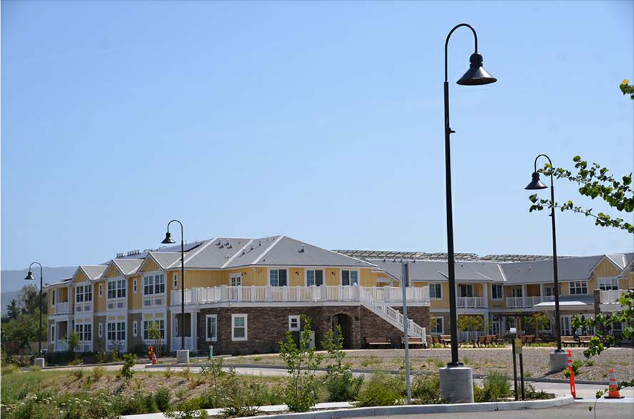
AS BUILT 20 FOOT TALL LIGHTS
