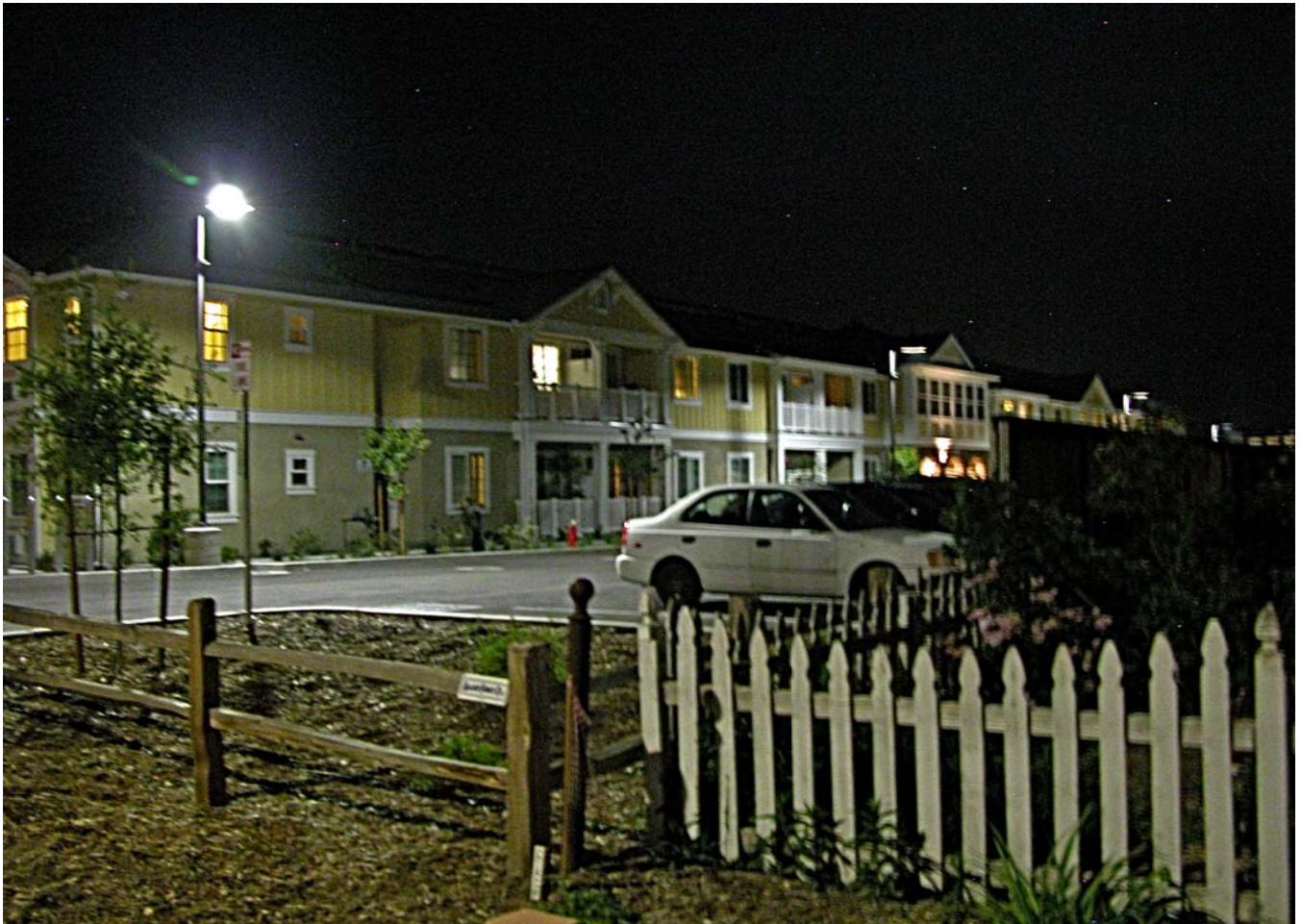
AS BUILT 20 FOOT TALL LIGHTS
