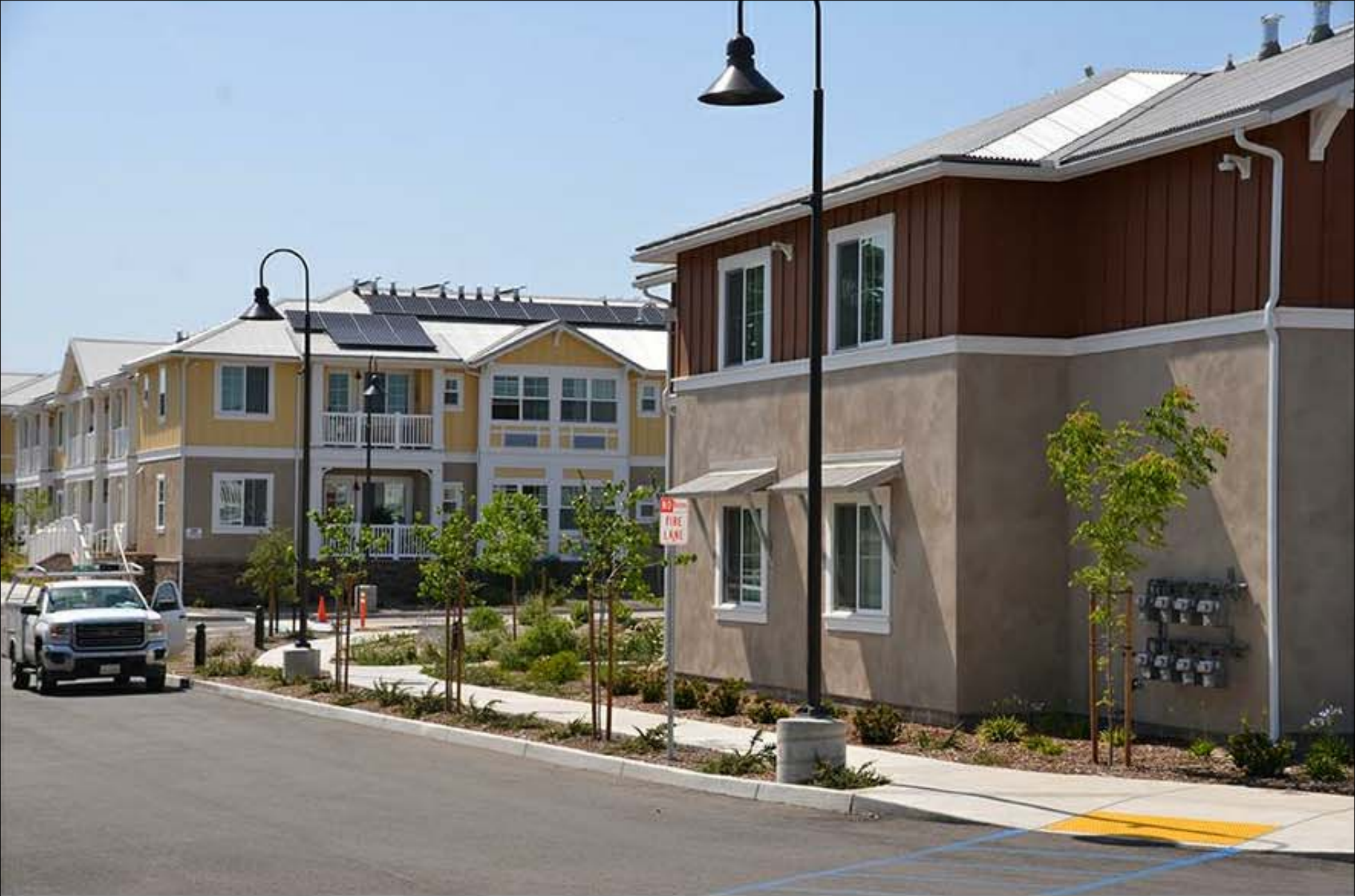
AS BUILT 20 FOOT TALL LIGHTS
