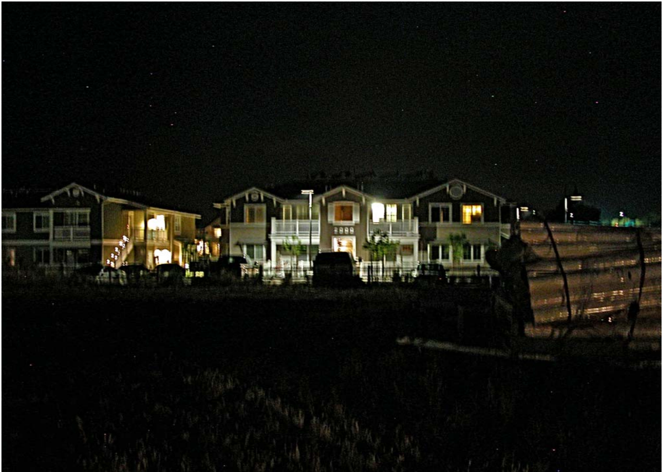
AS BUILT 20 FOOT TALL LIGHTS
