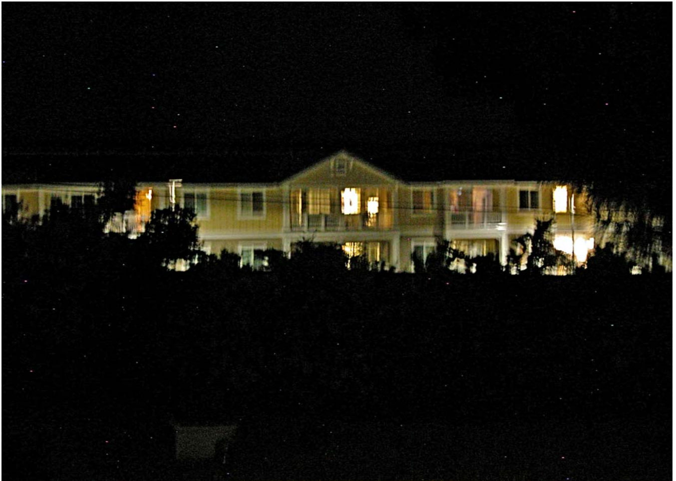
AS BUILT 20 FOOT TALL LIGHTS
