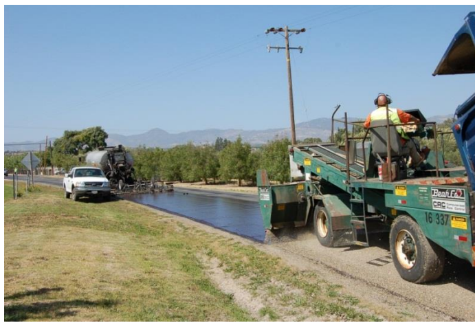
Typical scrub seal operation
