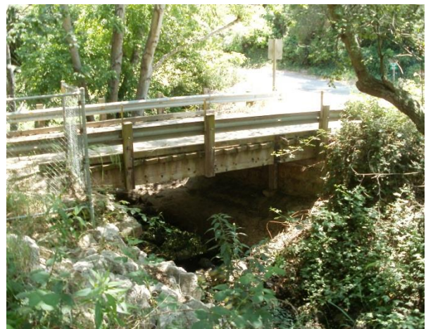
Western side creek bank view downstream
