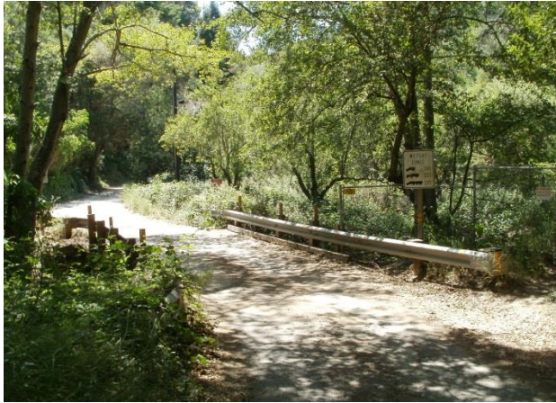
Eastern approach to Bridge 51C-214
