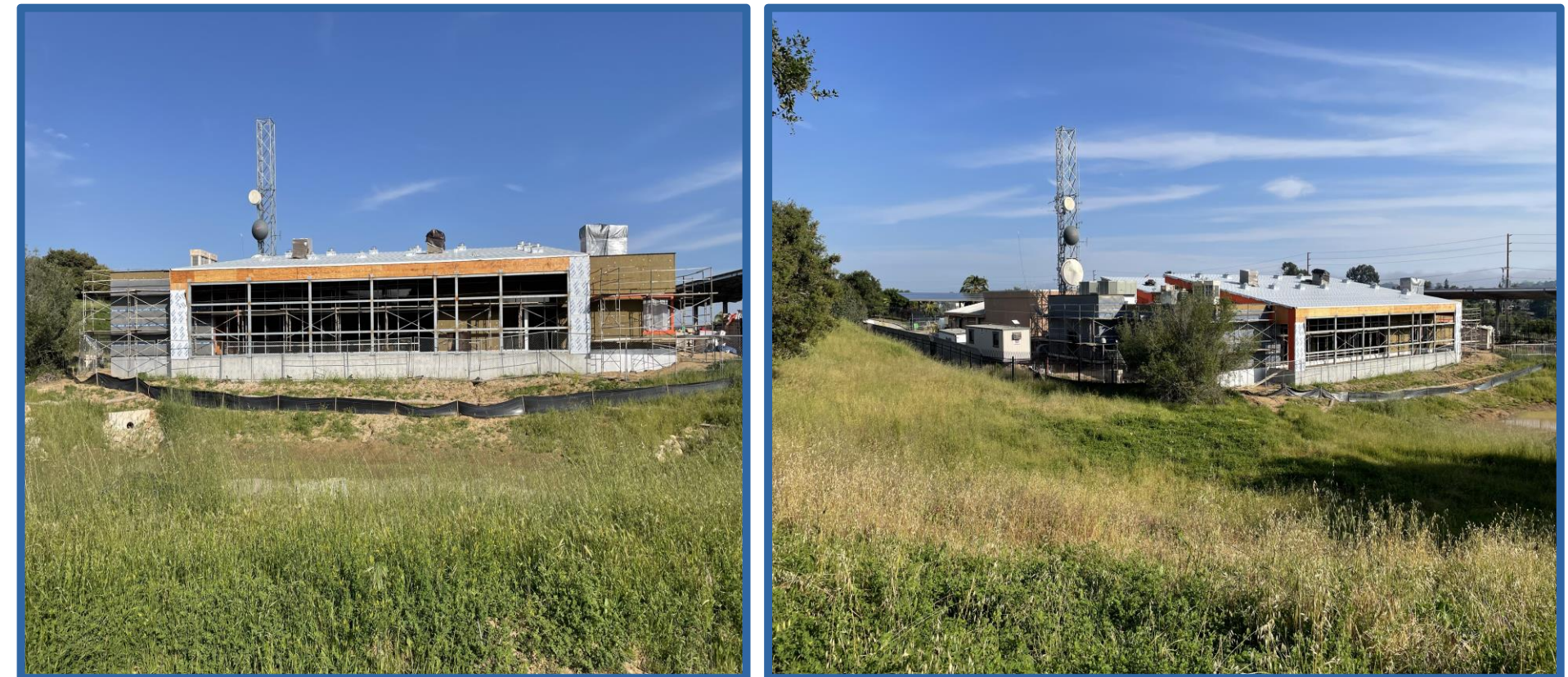
Fire Dispatch Center
