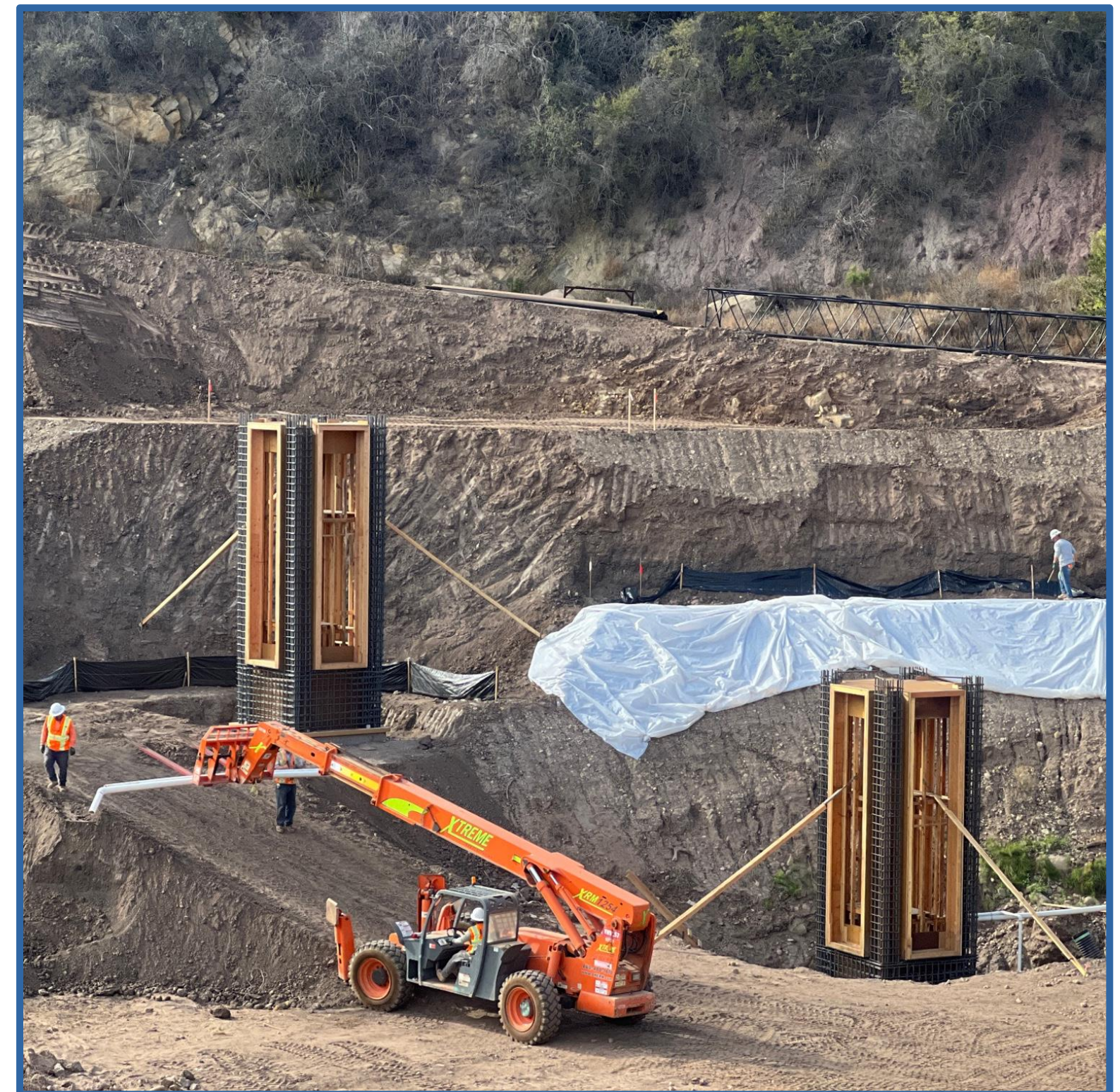
Santa Monica Debris Basin
