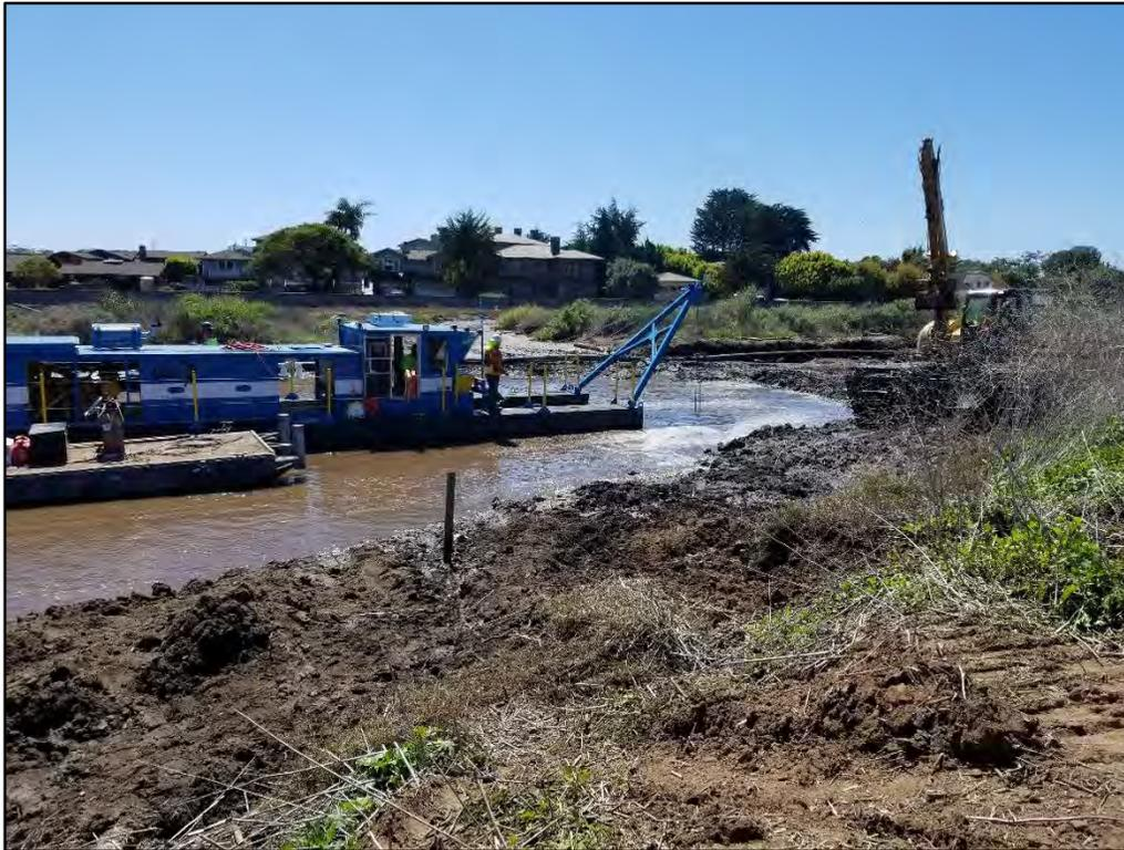
**Figure 4-3. Hydraulic Dredging Operation at the Marsh**
