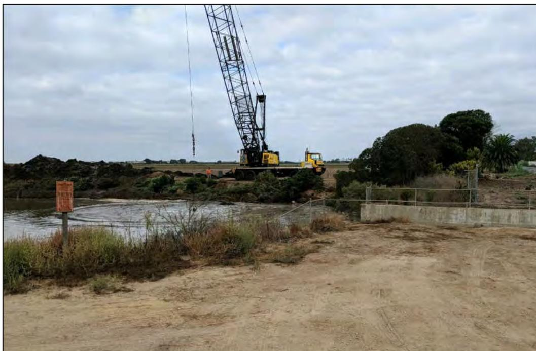
**Figure 3-5. Drag-line Desilting Operation on Santa Monica Creek**
