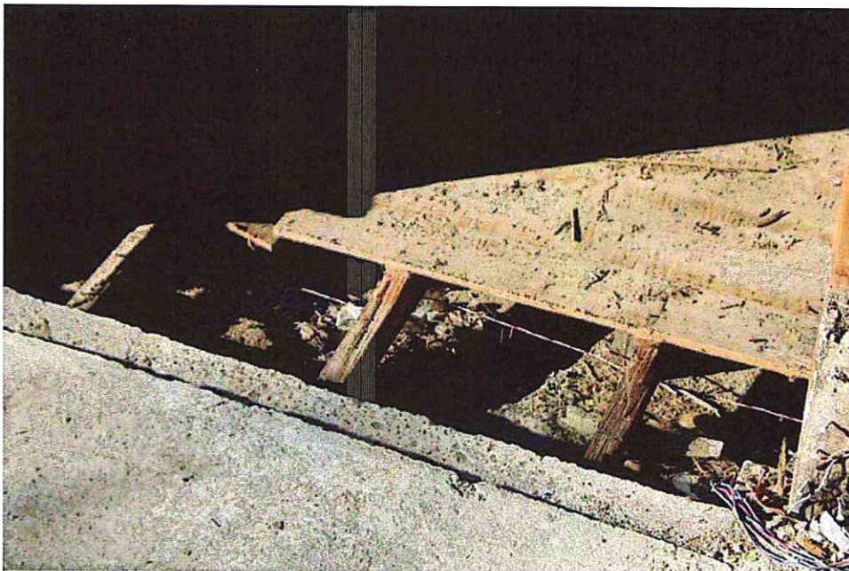
Photo 12: Rot at Floor Framing joists
