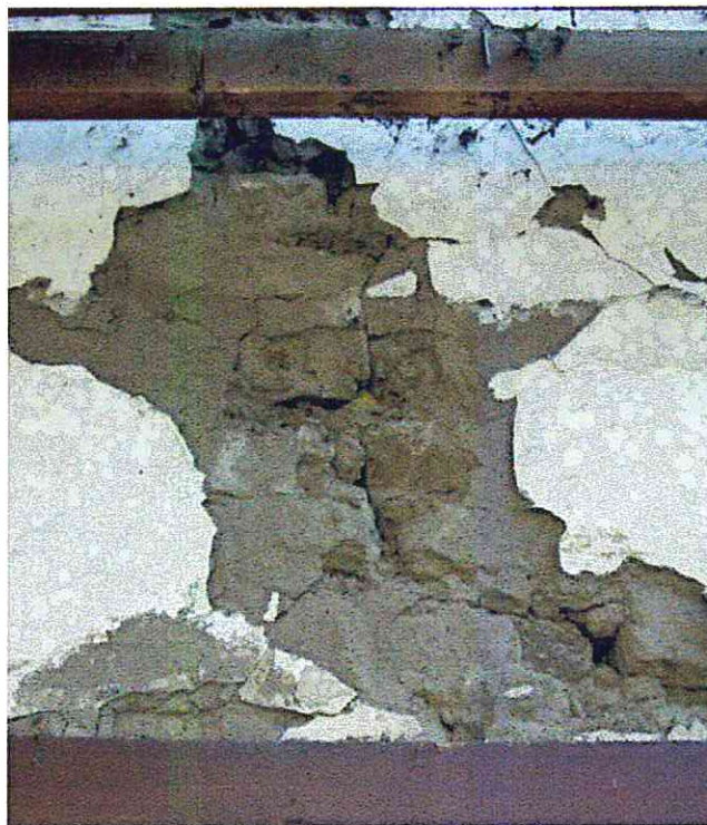
Photo 2 : Area of Wall where mortar and adobe brick are indiscernible
