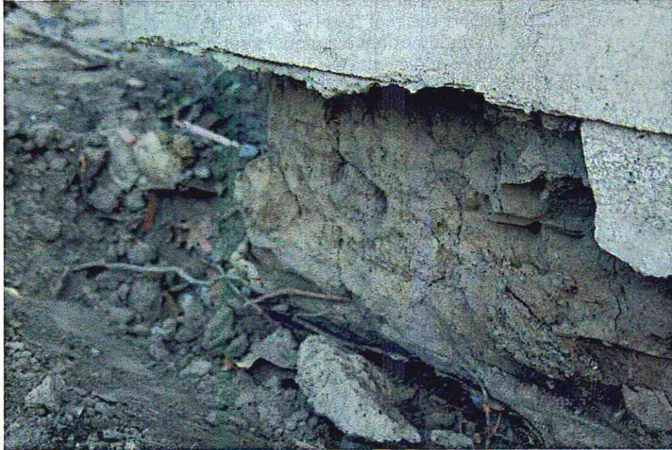
Photo 2 : Area of Wall where mortar and adobe brick are indiscernible
