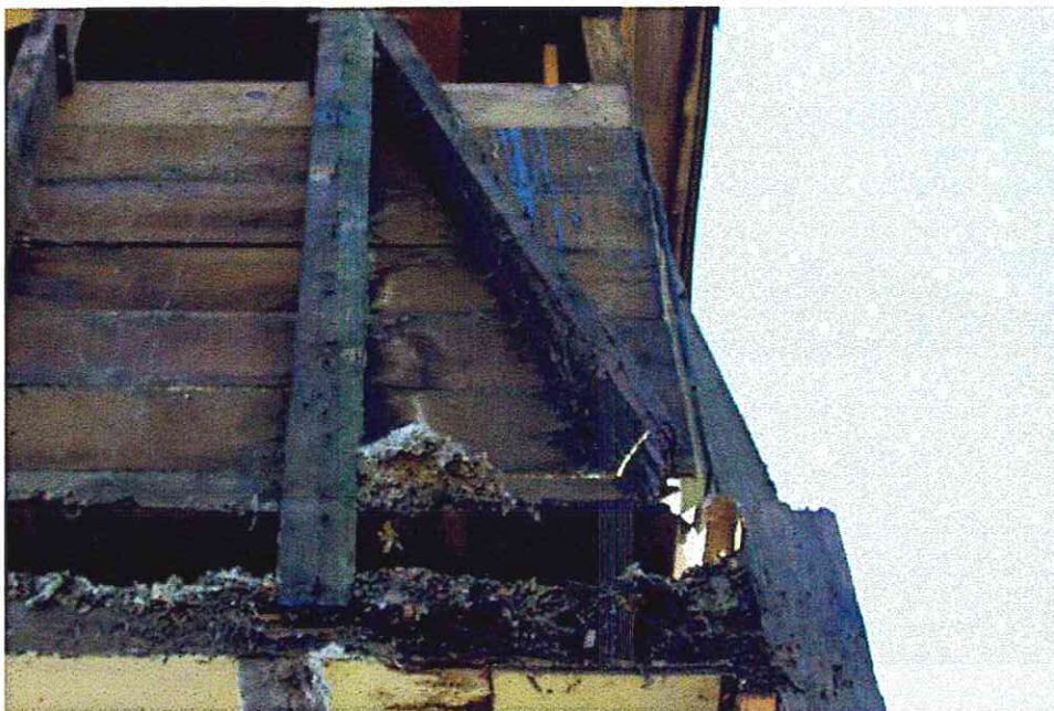
Photo 6 : Rot at upper floor where cross bracing meets floor plate. Corner post completely gone.
