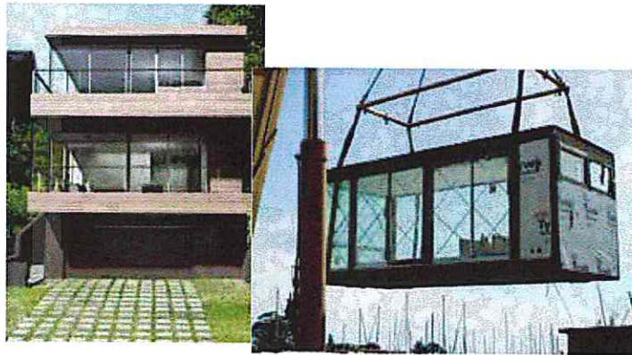
Fairview Modular Project, Santa Cruz, CA Architect: Marmol Radziner, Los Angeles, CA
