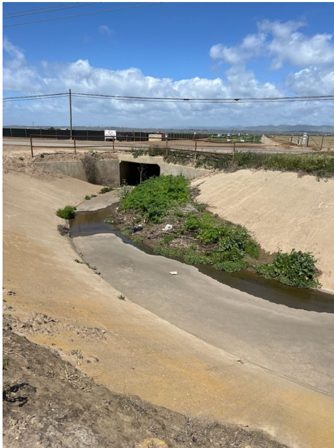
Unit 2 West Main Channel Section 2
