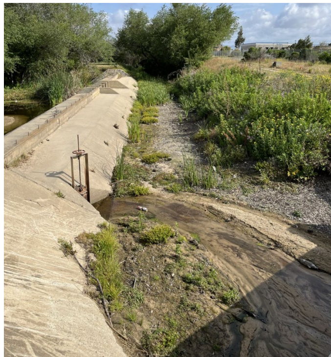
Santa Maria Airport Ditch Section 1
