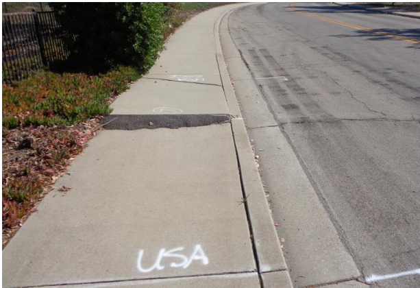
Before – Hummel Drive looking south
