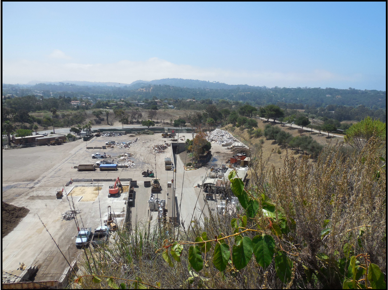
Exhibit 19: Photograph Overview Alternative 3 Site, SCRTS, View SSE
