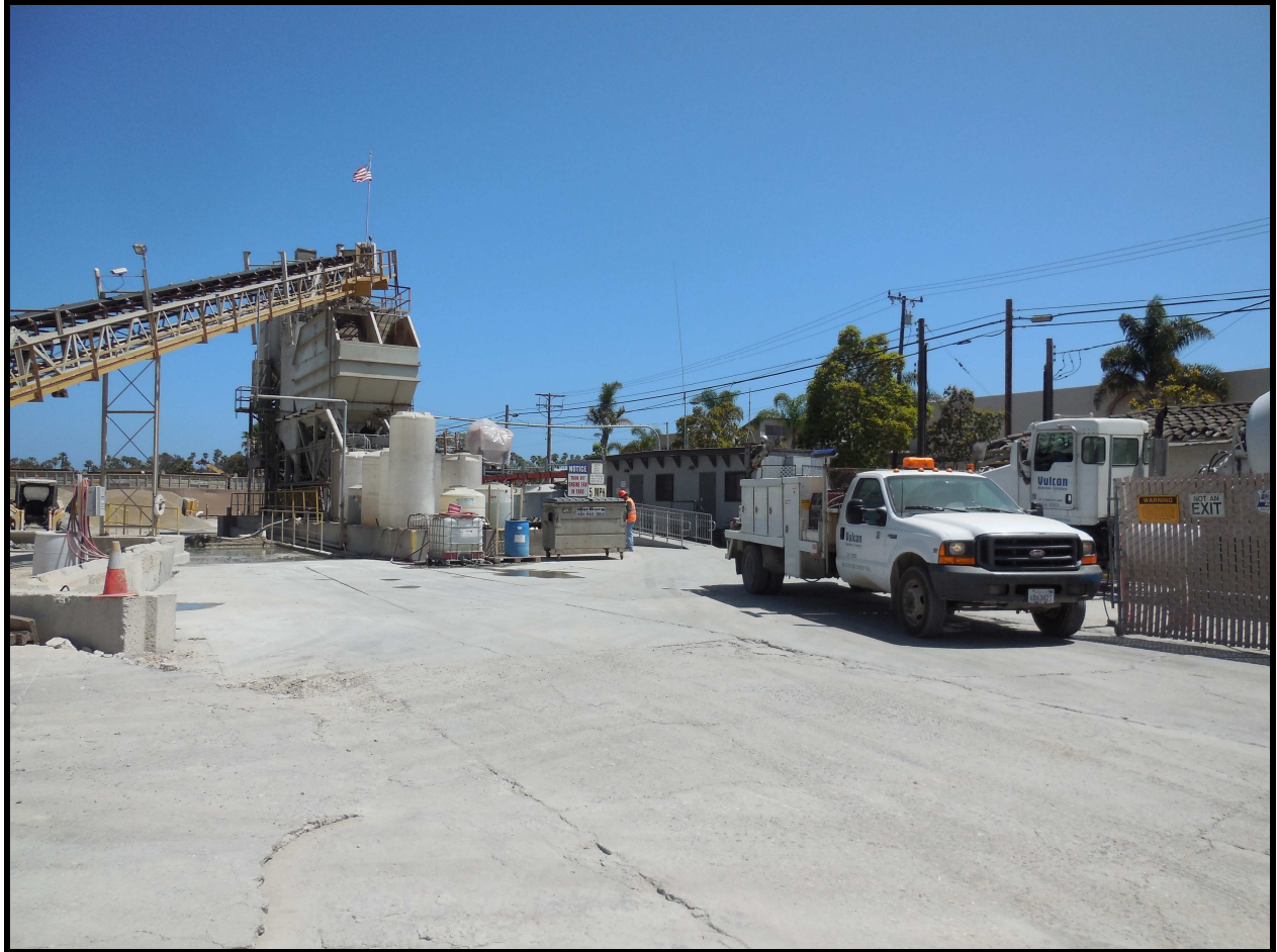
Exhibit 17: Photograph Overview Alternative 2 Site, 3 S. Calle Cesar Chavez, Santa Barbara, View South.
