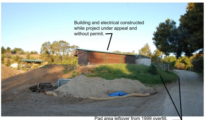
Further raised with fill dirt while under appeal and prior to construction of buildings. slope intersects right away without drainage and erosion control which causes road damage during heavy rains
