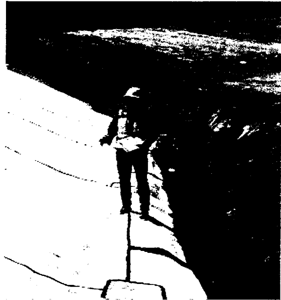
Geosyntec's CQA Monitor documenting geosynthetic repairs during construction of Tajiguas Phase IIIE Groundwater Protection System.
