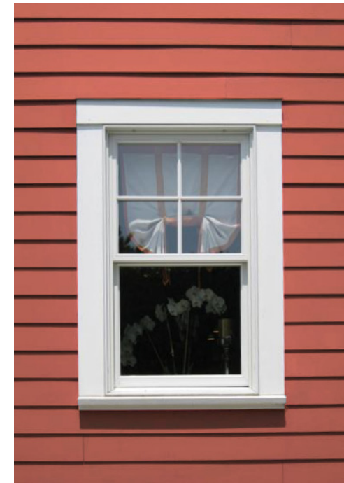
Figure 6.1 – Positive example of Window Relief, Wooden Siding, and Trim Detail
