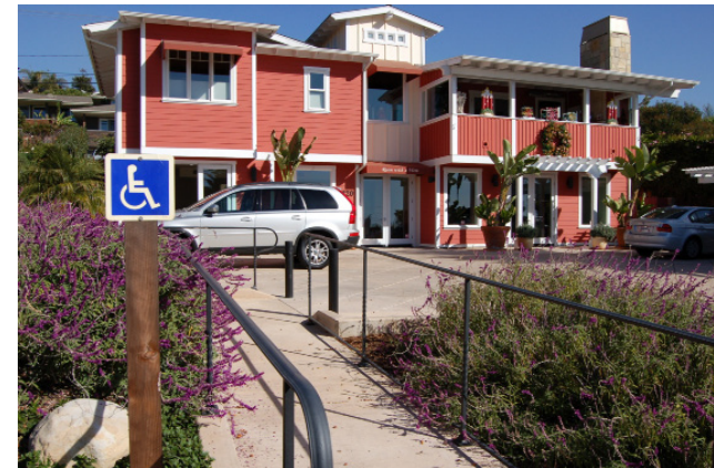
Figure 3.6 – Compatible ADA Ramp Example
