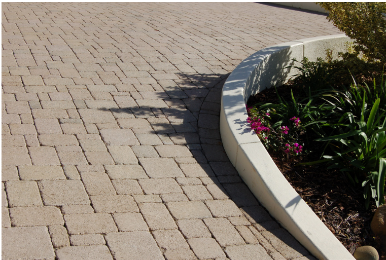
Figure 7.4 – Example of Permeable Pavers
