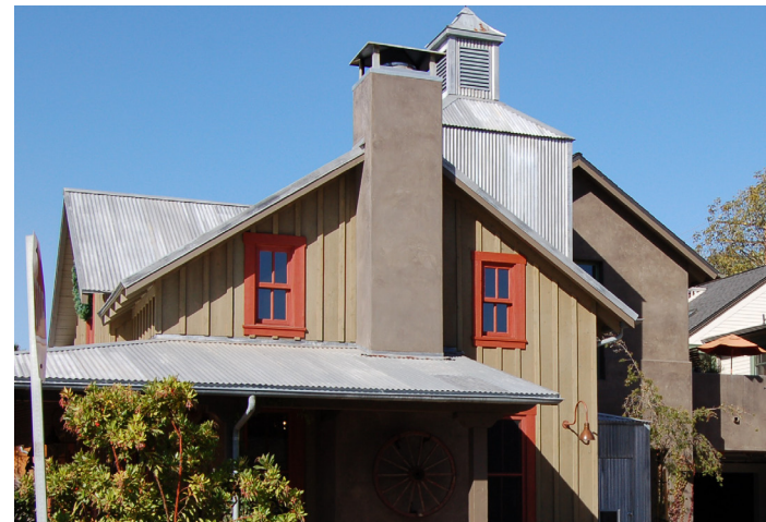
Figure 5.9 – Example of Varied Roof Elements
