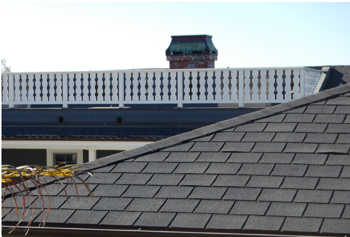
Figure 5.8 – Roof Example with Hidden Rooftop Equipment
