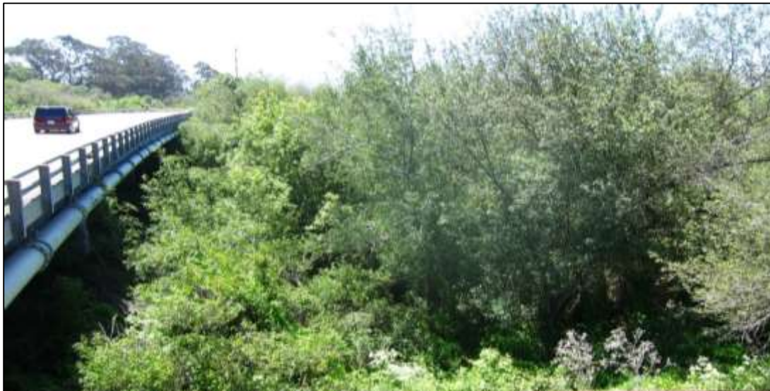
Existing Floradale Avenue Br. No. 51C-006 over the Santa Ynez River, view east
