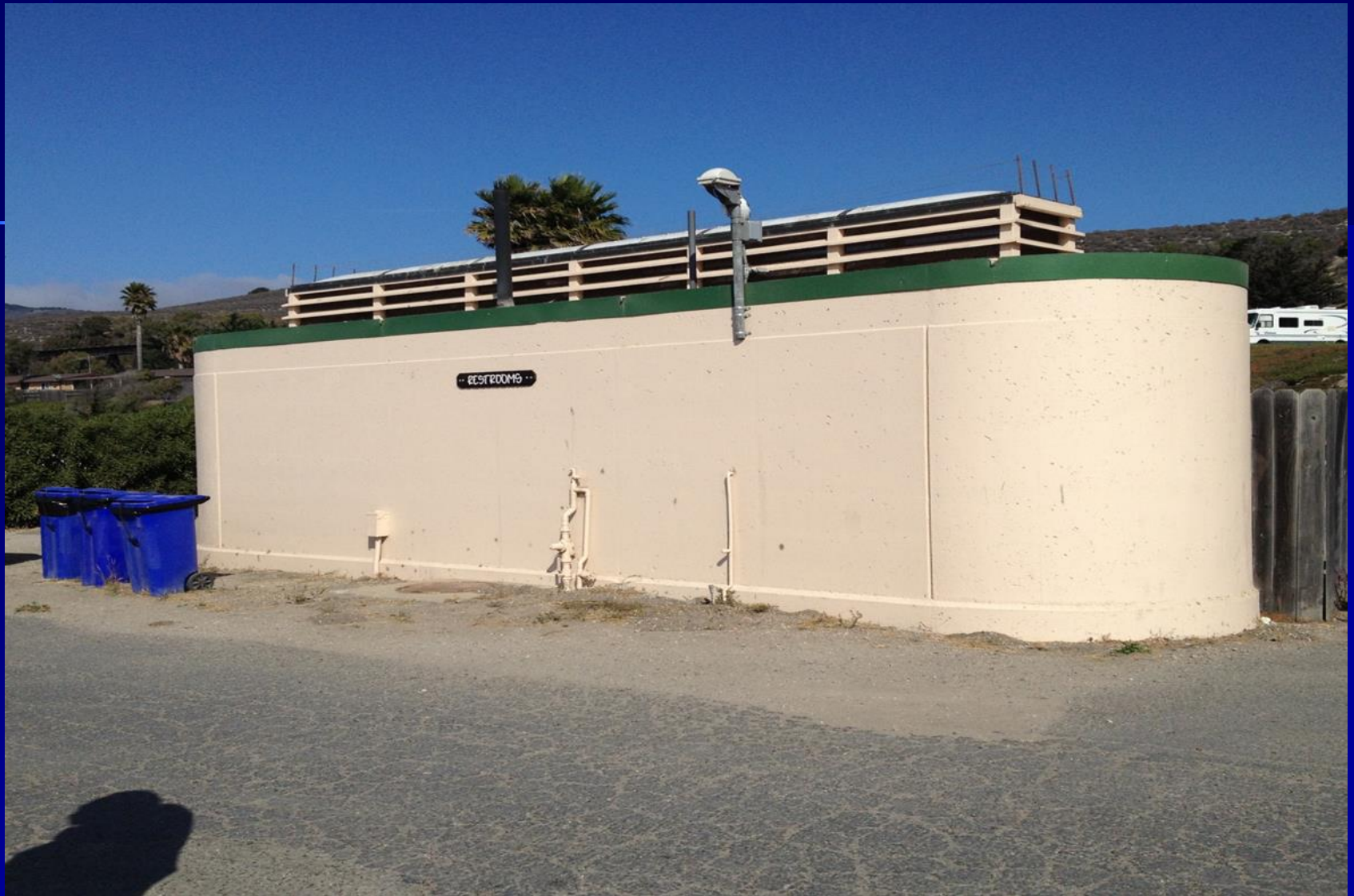
EXISTING LARGE RESTROOM – PROPOSED TO BE REPLACED
