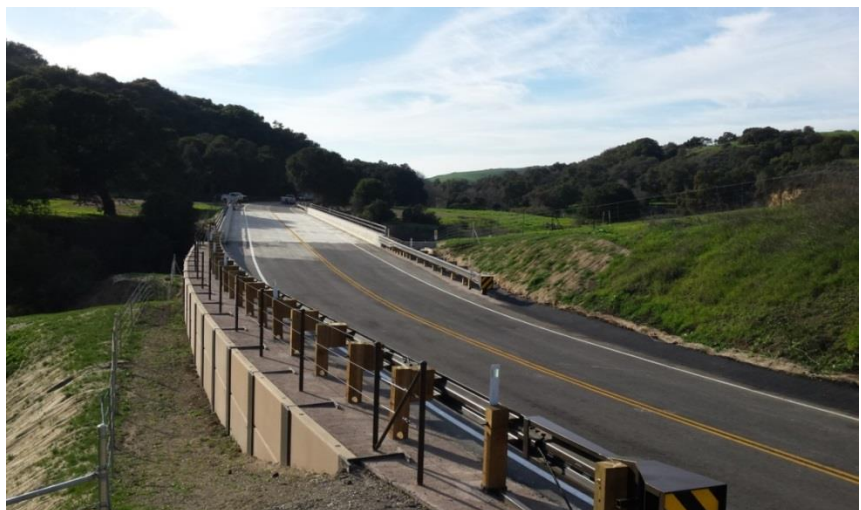
Post-Construction – Looking west, northwest on February 12, 2016
