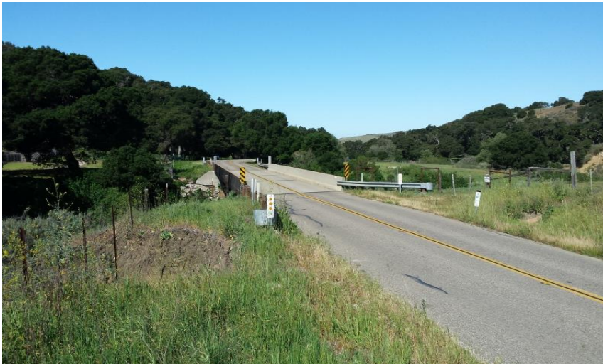
Pre-construction Bridge - Looking west, northwest on March 27, 2015
