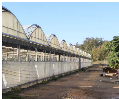
Figure 2- Existing Greenhouse 1 Exterior
