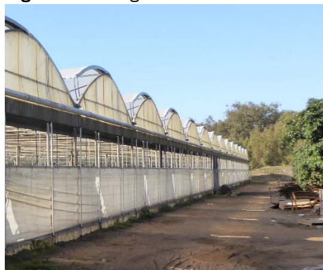
Figure 4- Existing Greenhouse 1 Exterior
