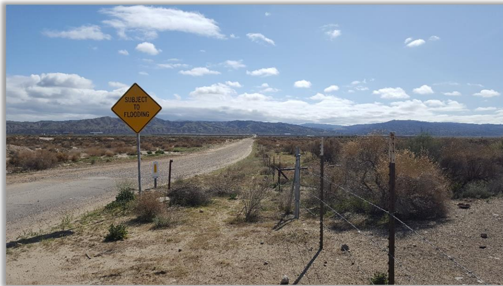
Foothill Road Low Water Crossing – Looking East
