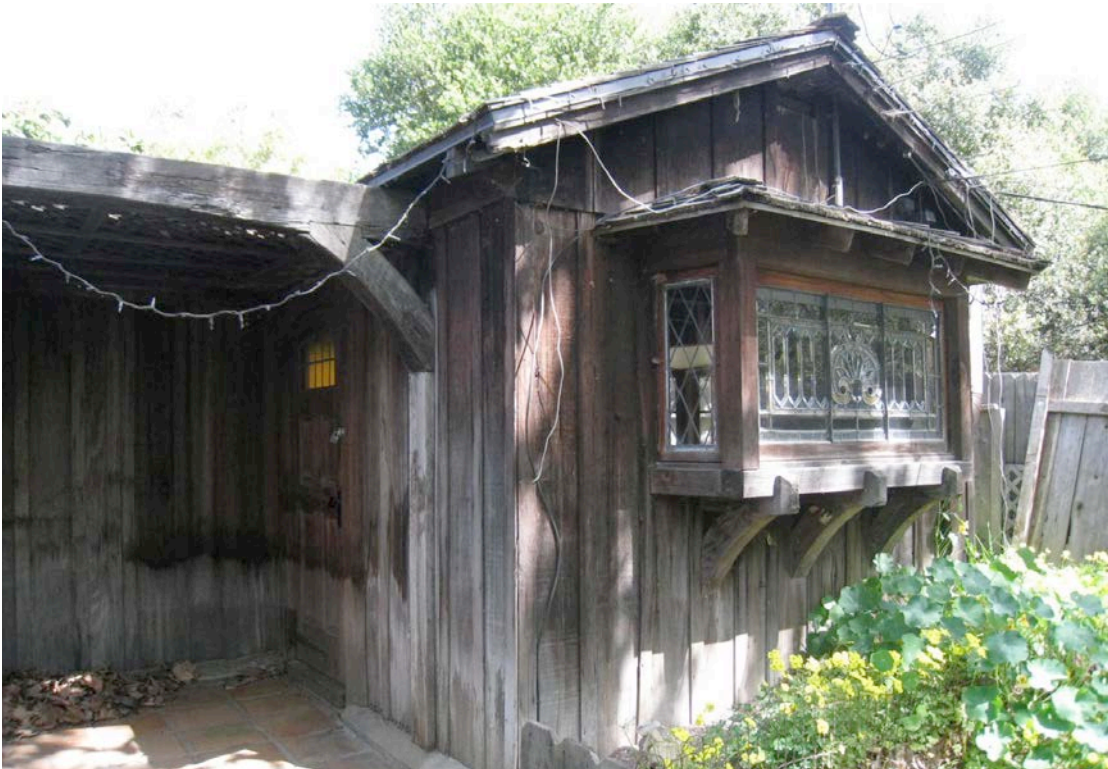
Plate 21. Cottage. South elevation showing recessed porch area to be replaced with storage addition. Facing north. April 2010. A. C. Cole
