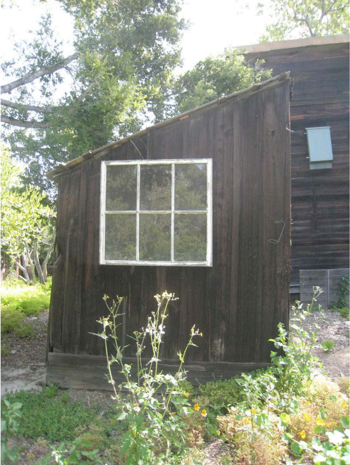
Plate 17. Detail of west elevation of west shed-roof lean-to showing relationship to water tower at rear. Facing east. April 2010. A. C. Cole
