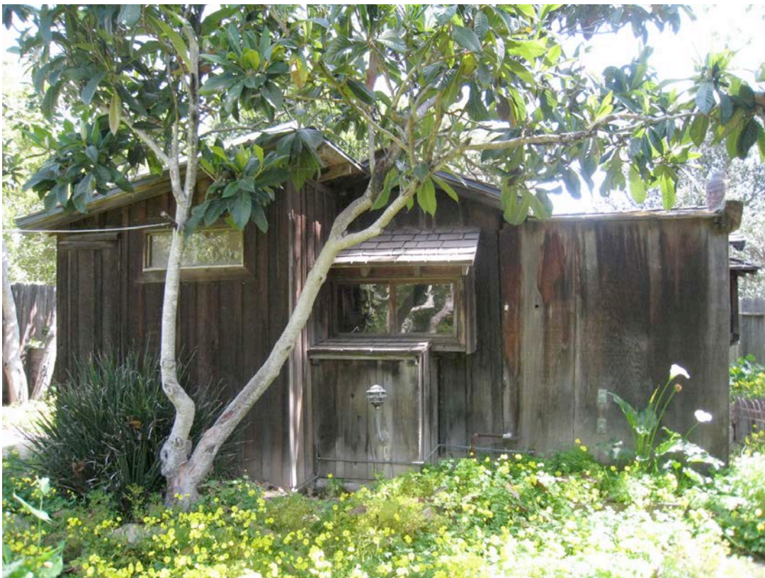
Plate 23. Cottage. North elevation. Facing south. April 2010. A. C. Cole
