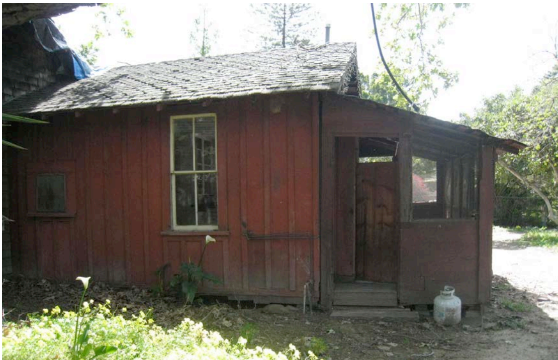
Plate 4. North side of kitchen wing. Lean-to at right to be replaced with a gabled extension and paired 2/2 pane windows to be added. Facing south. April 2010. A. C. Cole
