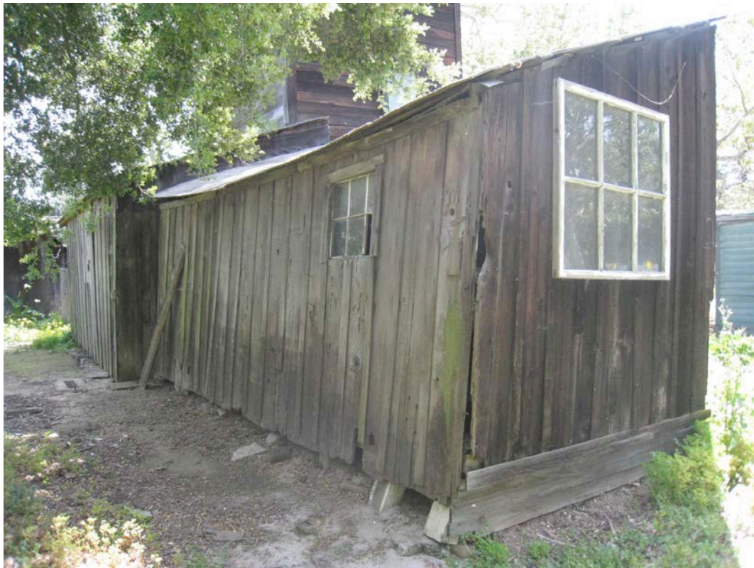
Plate 16. Detail of north and west elevations of north and west shed-roof lean to wings to water tower to have 2/2 pane windows added. Facing southeast. April 2010. A. C. Cole
