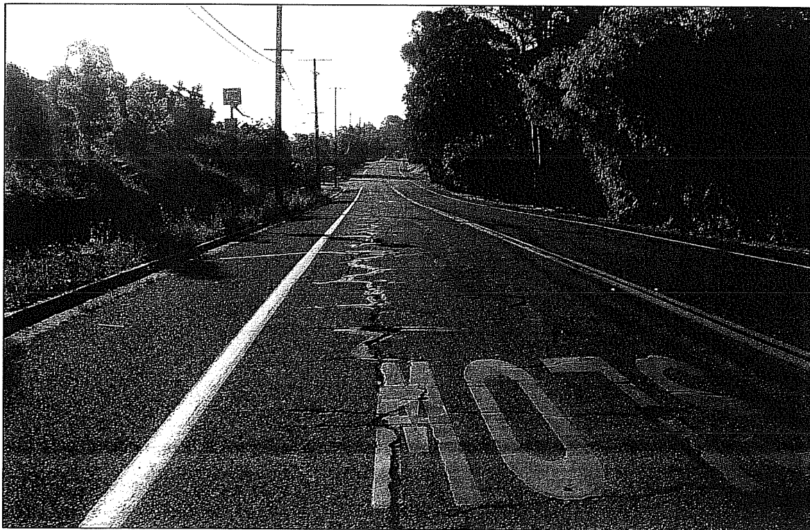
Typical site to be rehabilitated - Modoc Road
