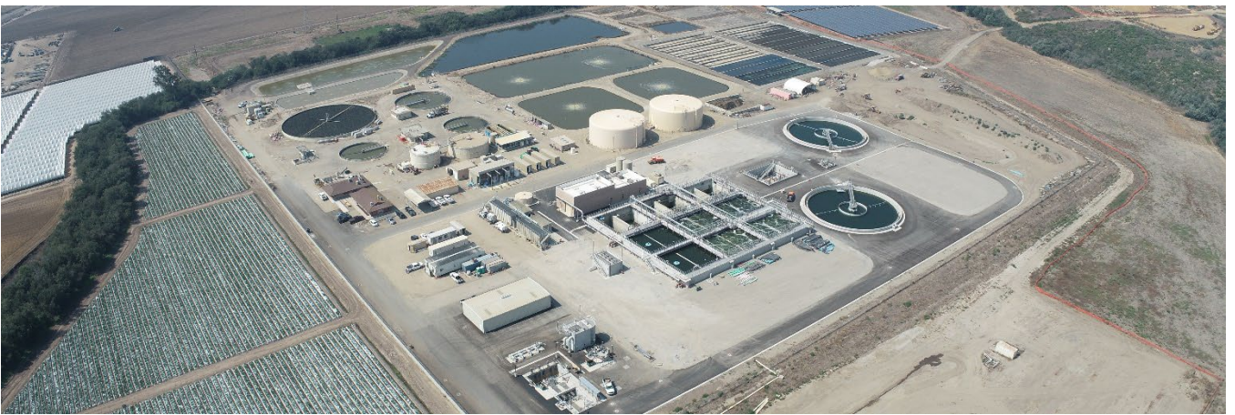
Recently Upgraded Laguna County Sanitation District Wastewater Treatment Facility
