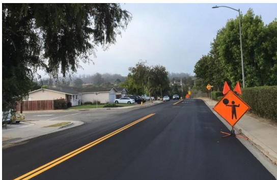
Fourth District – Orcutt Frontage Road
