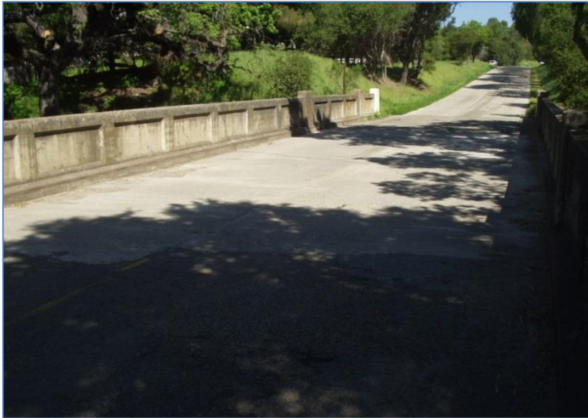
Old Jonata Park Road Bridge No. 51C-226
