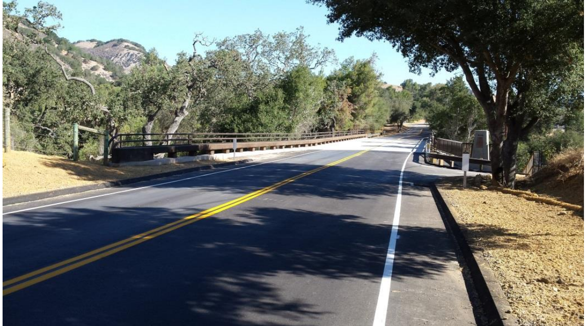
New Jonata Bridge 51C-0356 Looking North
