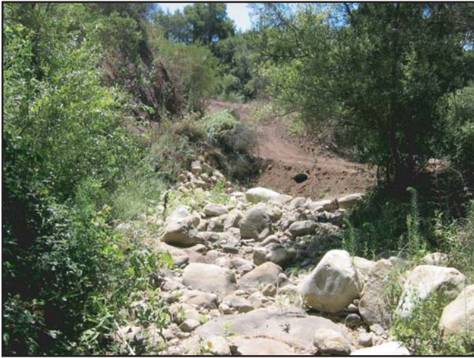
Photo 1 - South-facing view of Sutton Canyon (see Figure 1), current conditions.
