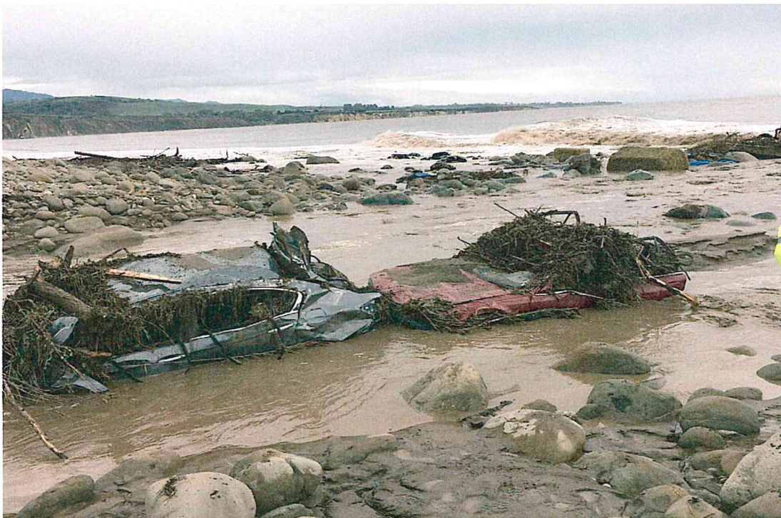
Figure 9 : Twisted metal I-beams which supported a bridge prior to the debris flow event
