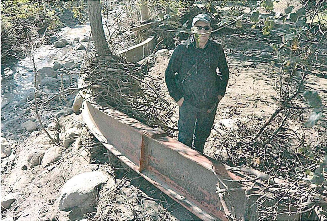
Figure 9 : Twisted metal I-beams which supported a bridge prior to the debris flow event
