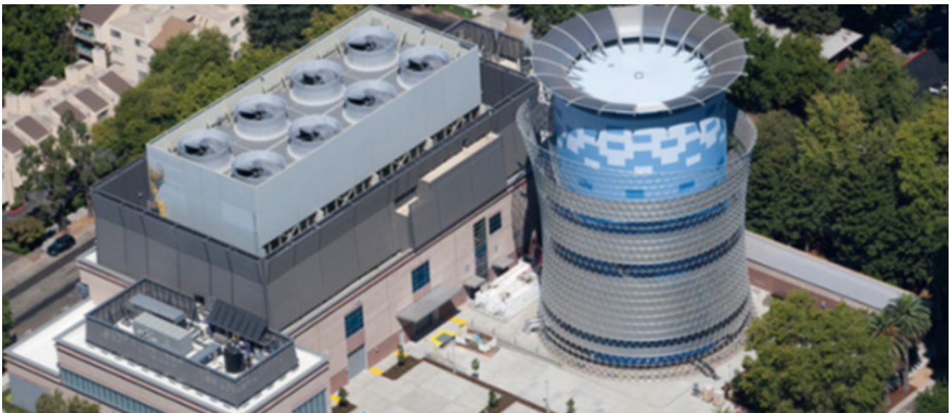
California Department of General Services, Sacramento Central Utility Plant
