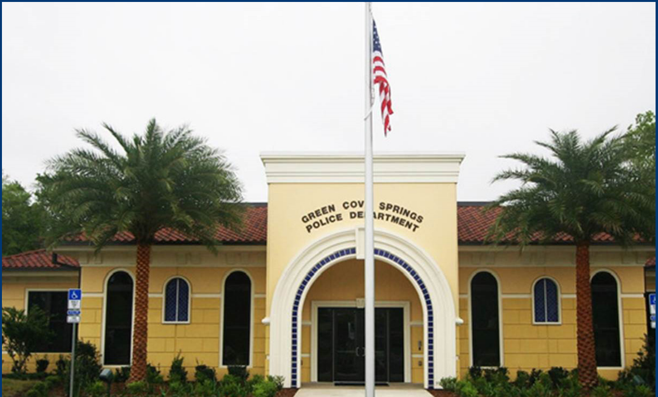
Green Cove Springs, Public Safety & Emergency Operations Center, FL
