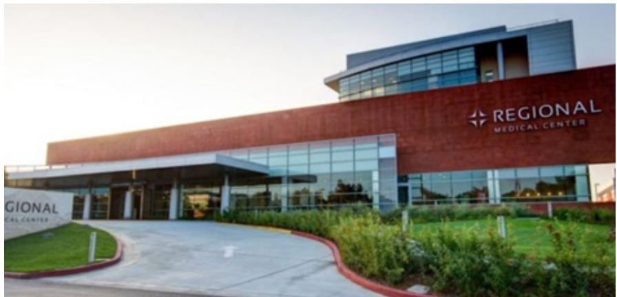
Regional Medical Center of San Jose, 4-Story Patient Wing Addition
