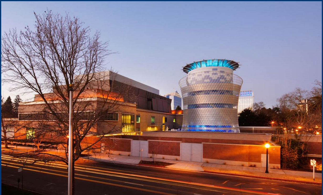
State of California Central Utility Plant, Sacramento, CA
