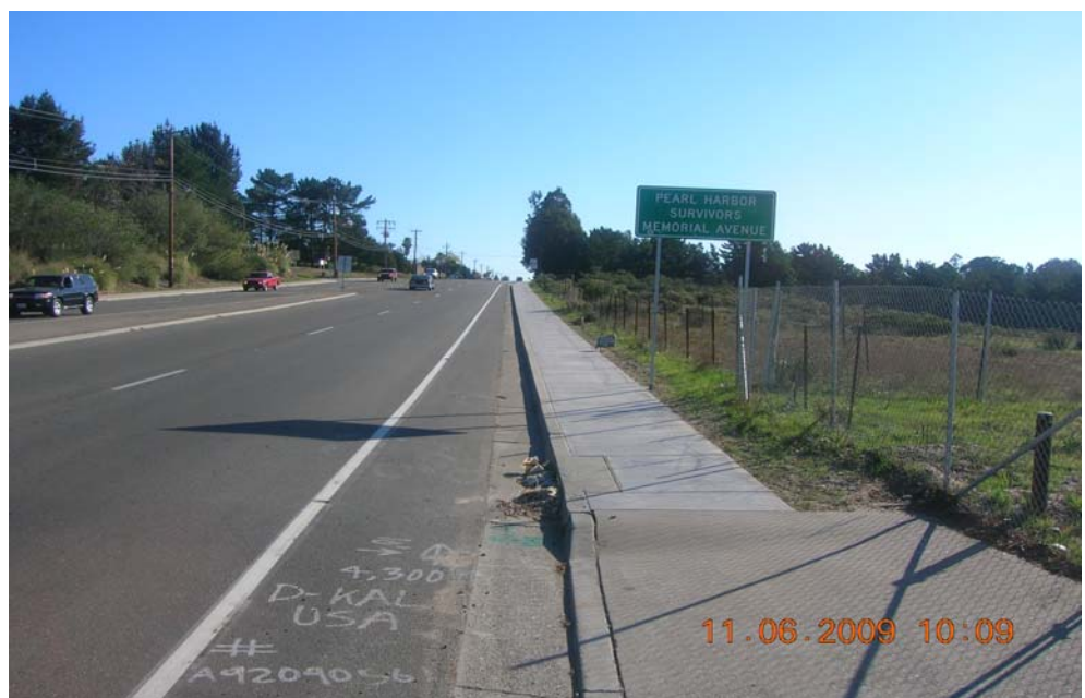
New Sidewalk on Clark Avenue in Orcutt
