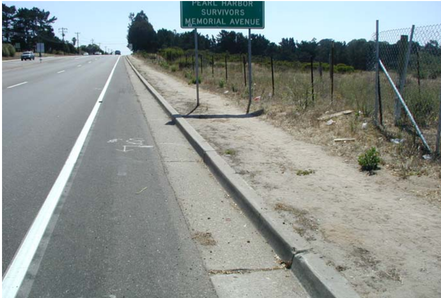
Clark Avenue in Orcutt prior to Construction
