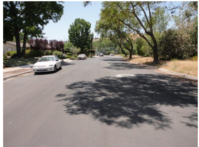
Via Regina – Completed
