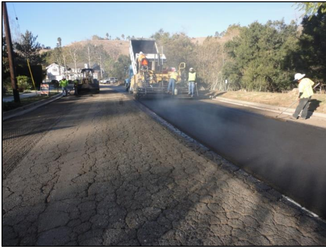
Paving on Via Regina
