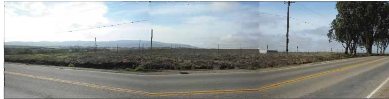
WEST VIEW #2 AT BLACK ROAD SOUTH OF BETTERAVIA ROAD
