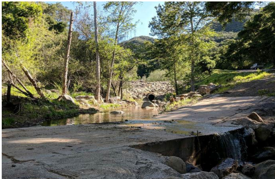
Photograph 4.5-2: Maria Ygnacio Creek, Main Branch Debris Basin Looking Upstream; Pre-project
