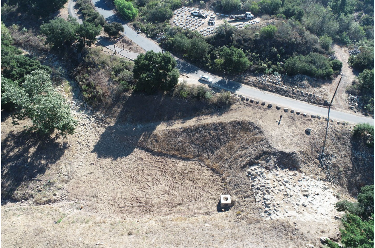
Photograph 5.1-1: Arroyo Paredon Creek Debris Basin
