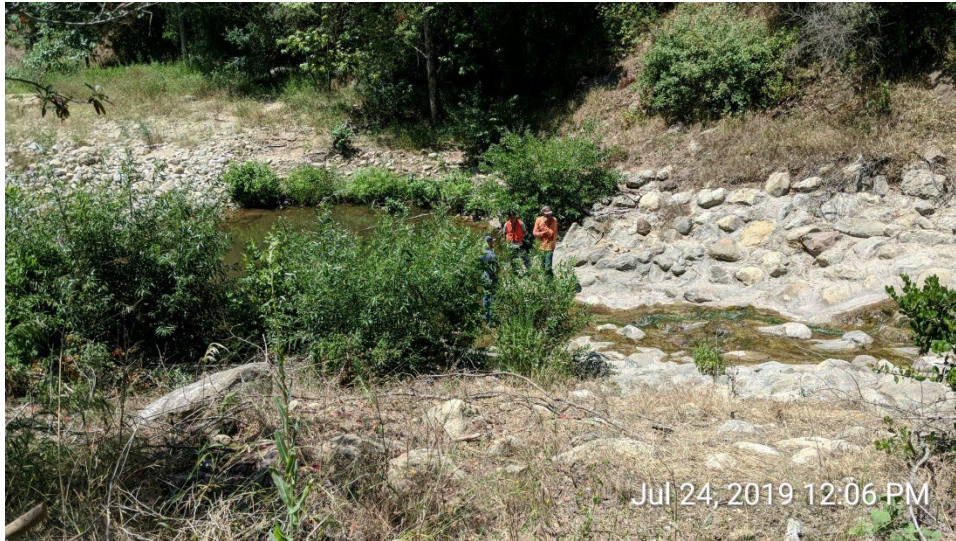
Photograph 4.5-1: Maria Ygnacio Creek, Main Branch Debris Basin Inlet Structure; Pre-project
