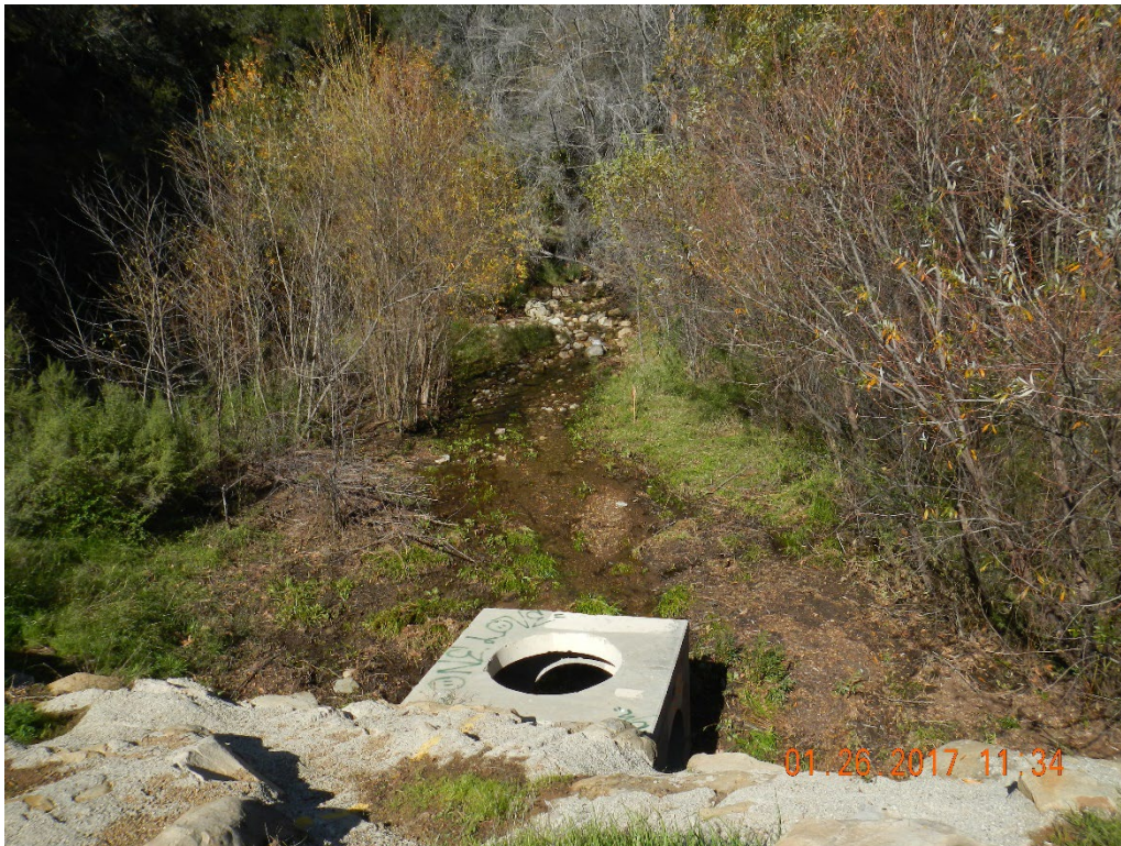
Photograph 5.3-2: Rattlesnake Creek Debris Basin
