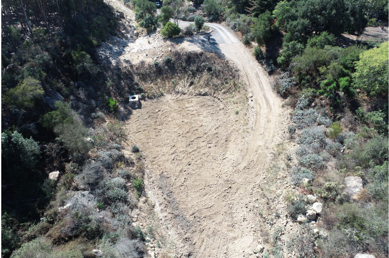
Photograph 6.7-1: Upper West Toro Canyon Creek Debris Basin
