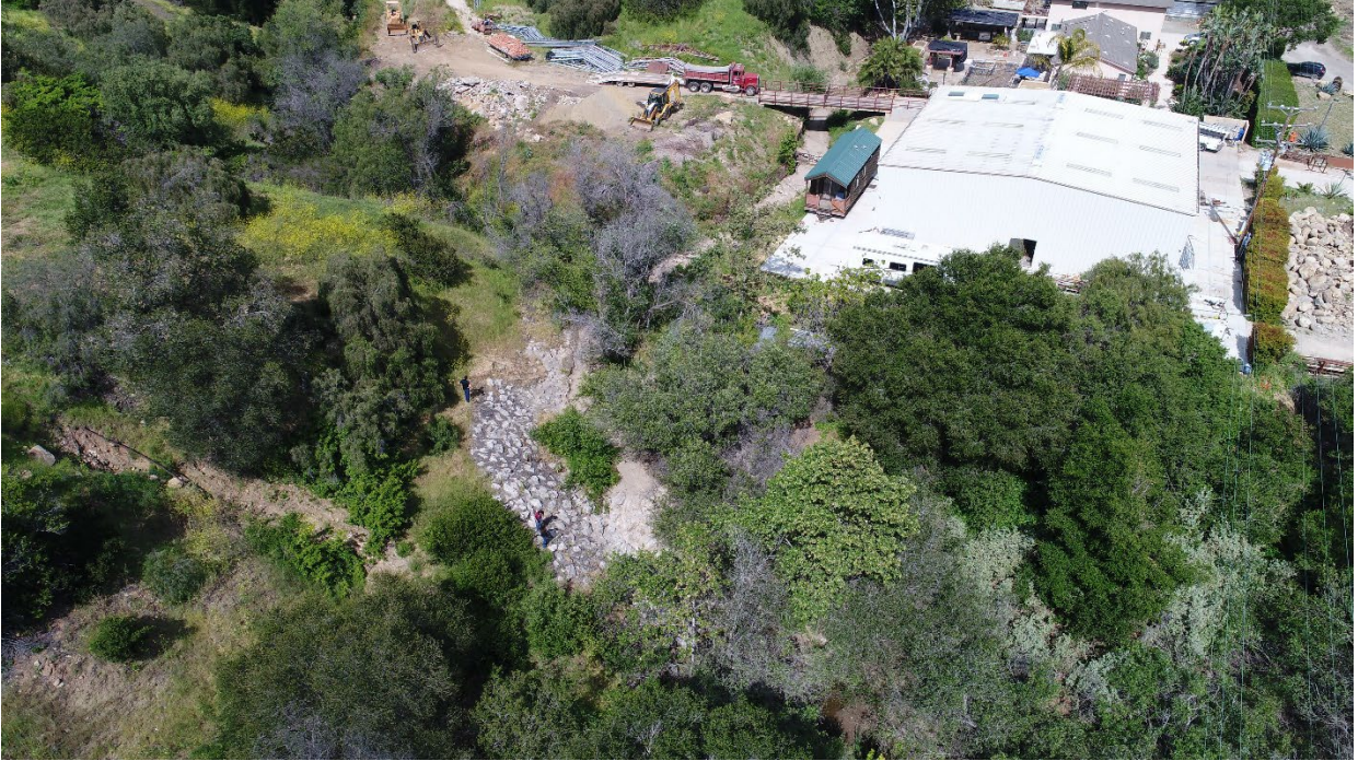
Photograph 4.4-1: Maria Ygnacio Creek, East Branch Debris Basin Upstream
