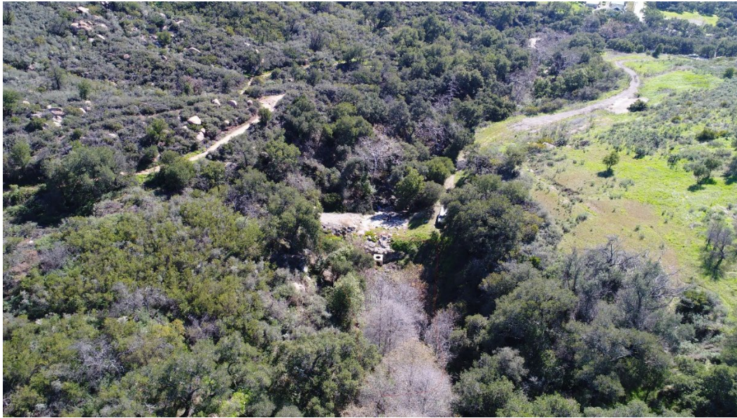
Photograph 5.3-1: Rattlesnake Creek Debris Basin
