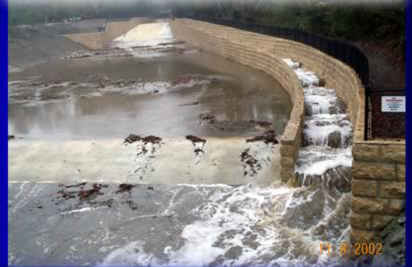
Montecito Creek Debris Basin
