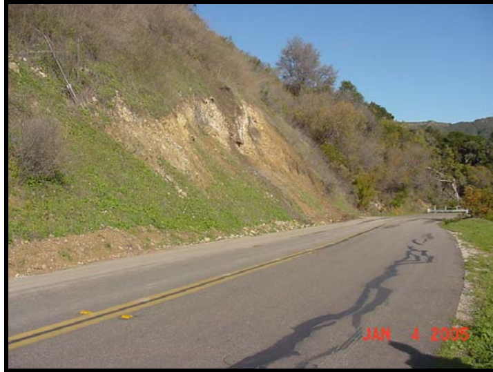
Photo: Existing Jalama Road embankment and roadway conditions
