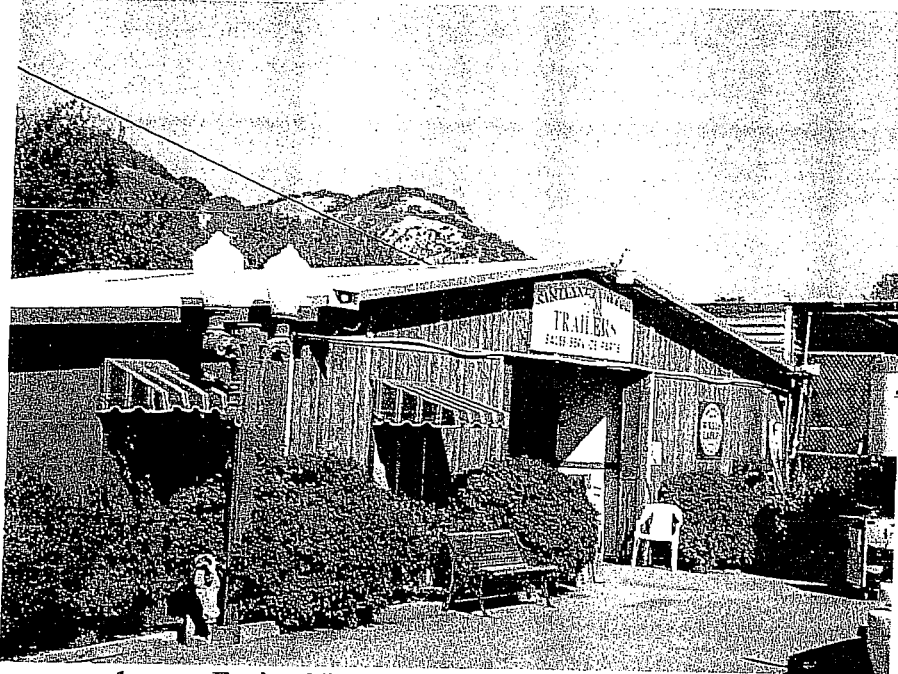
1. Facing North West from Trailer Sales Yard The top sign is ~3'6" x 8"; the right sign is ~3' x 3'.
