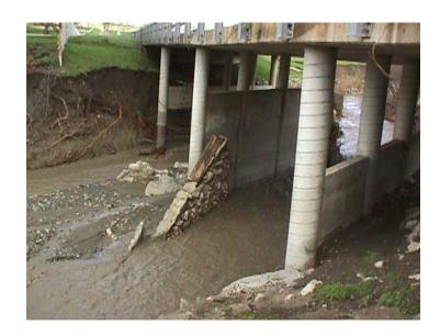
The project will stabilize the creek bottom beneath the Alisos Avenue Bridge by constructing a grade stabilization structure consisting of a cut-off wall 25 meters long at the upstream portion of the repairs. This cutoff wall will maintain a constant streambed elevation beneath the bridge.
