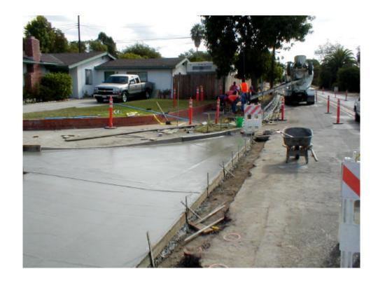
The project is one of the strategies the Department employs in its annual Preventive Maintenance Program and consists of repair of the existing hardscape by the removal and replacement of damaged concrete curbs, gutters and sidewalks, installation of federally mandated curb ramps, tree removal, tree root pruning and shielding. Approximately 5,278 linear feet of sidewalk and 4,237 linear feet of curb and gutter will be repaired with the construction of this project.
