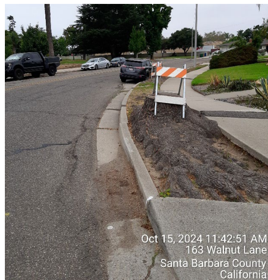
Figure 2: Typical Location of Hardscape repairs - Walnut Ln
