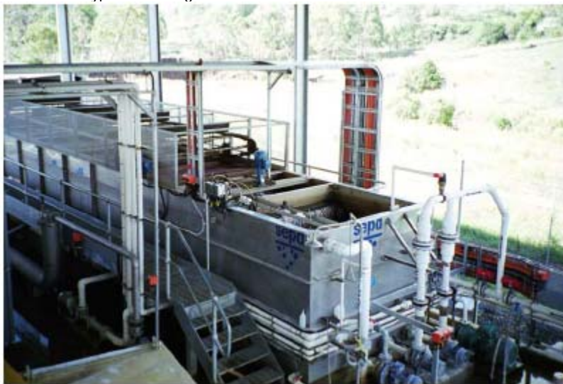
FIGURE 3-8 Picture of a Typical Rectangular DAFT
