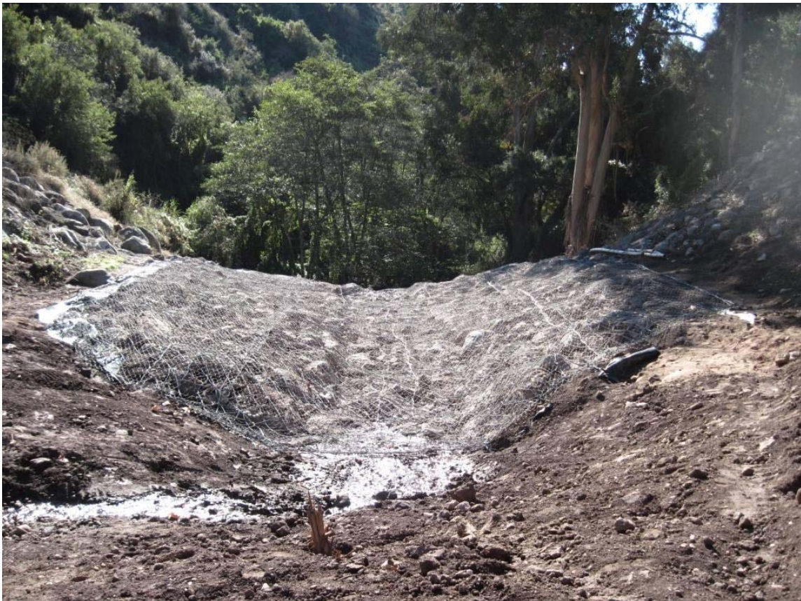
Lillingston Canyon Debris Basin Phase 1 Removal Project Completion
