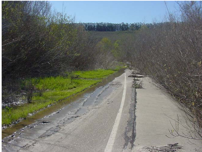
Existing Roadway March 4, 2004
