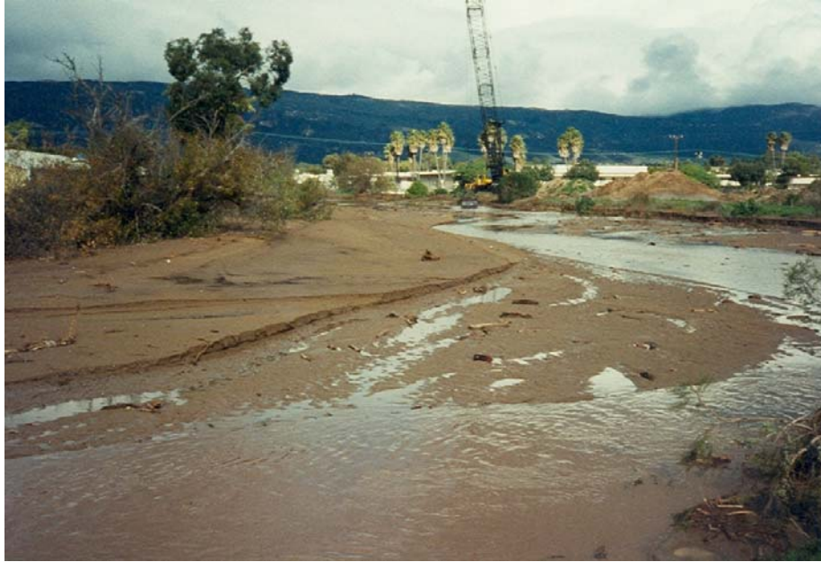
Figure 5 – Carneros Creek Sediment Basin, 1995
